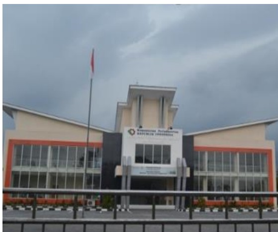
Figure 3. Front view of ATK Academy building
