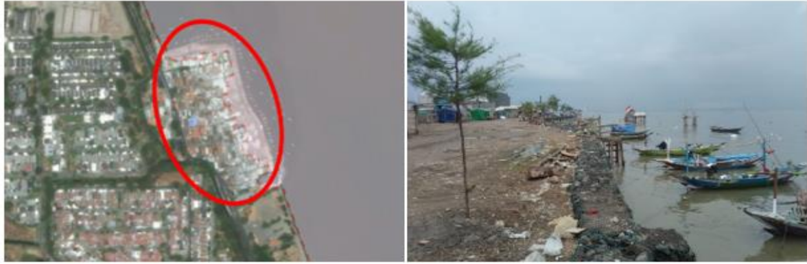
Figure 7. Reclamation and seawall at Kenjeran beach
