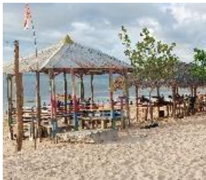
Figure 13. Condition of tourist facilities in Tablong Beach Area
