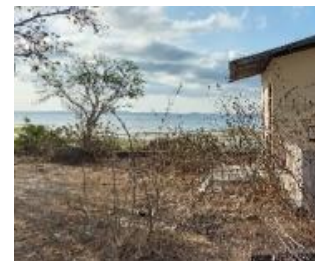
Figure 6. Condition of clean water facilities in Tabolong Beach Area
