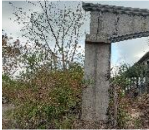
Figure 11. Abandoned hotel conditions in Tablong Beach Area
