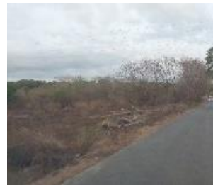
Figure 3. Road Conditions to Tabolong Beach Area
