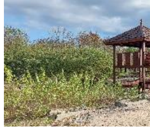
Figure 10. The condition of the gazebo in the Tablong Beach area
