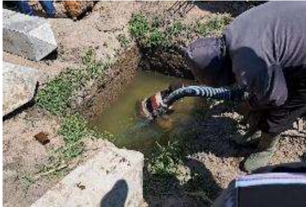
Gambar 4. Memompa air
