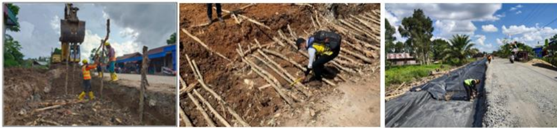
Figure 3. Soil Improvement used in Central Kalimantan
