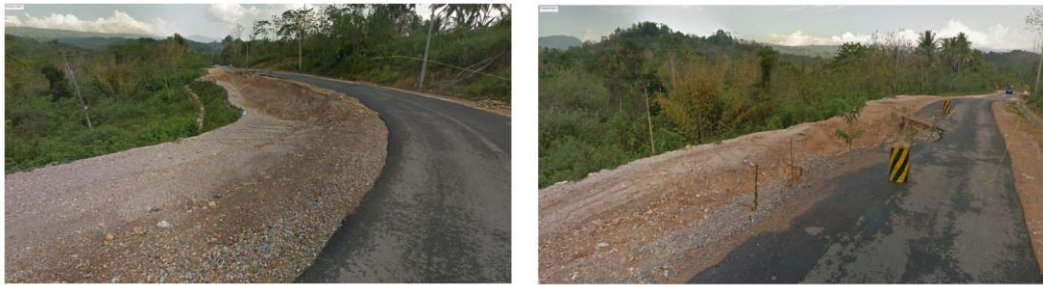
Figure 2. Slope before reinforcement (Satker PJN Wil. II Provinsi Sulawesi Tenggara, 2020)
