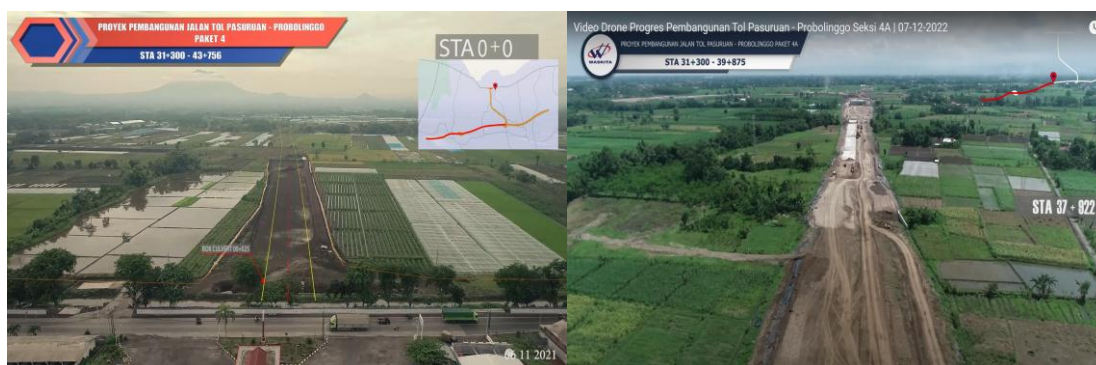
Figure 2. Condition of Pasuruan-Probolinggo Section 4 Toll Road (PT. Waskita Karya, Project Office)
