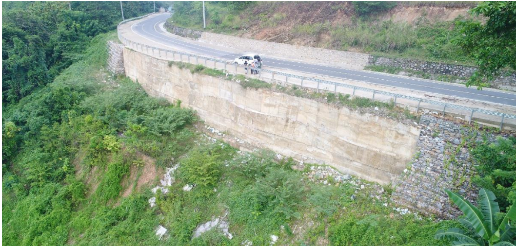
Figure 3. Condition of slope after the reinforcement
