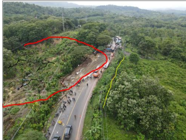
Figure 1. Slope Condition After Landslide Source: P2JN Aceh, 2023
