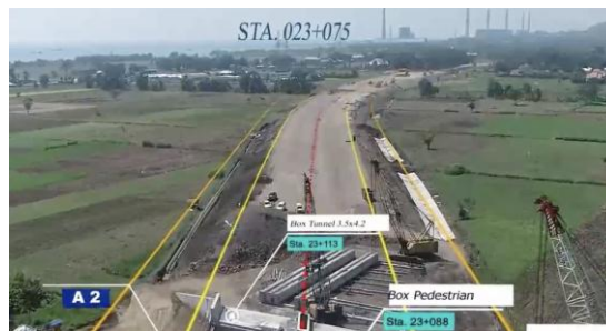
Figure 2. Location STA 23+075 (Source: PT Jasamarga Probolinggo Banyuwangi)
