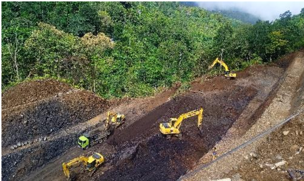
Figure 2. Implementation of excavation work
