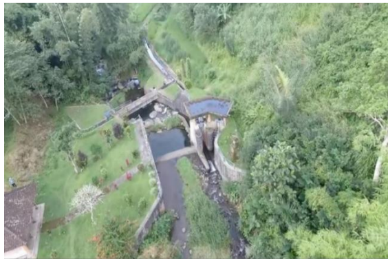
Figure 1. Weir and Primary Canal
