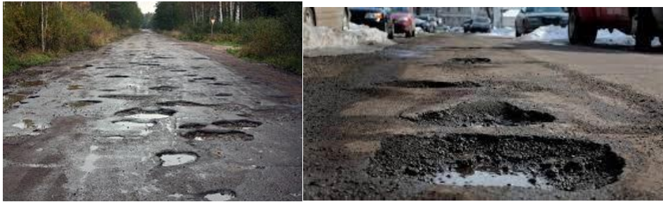
Figure 5. Road Potholes
