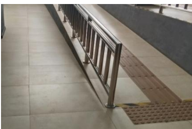
Gambar 4m. Ramp & Guiding Block
