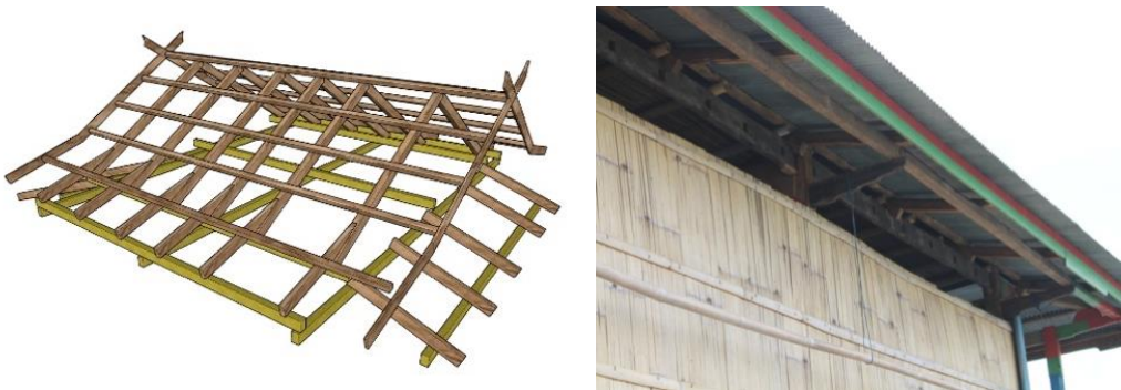
Figure 10. The Roof Tectonics of the Floating House is Lightly Exposed without a Ceiling. On the Front and Side
