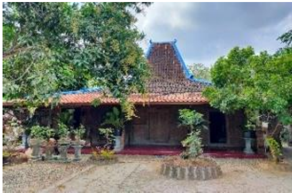
Figure 1. The Front View of Mr. Maryanto's House
