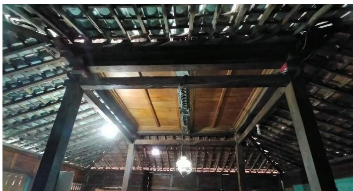
Figure 5. Usuk and Reng on the Roof Structure of the House
