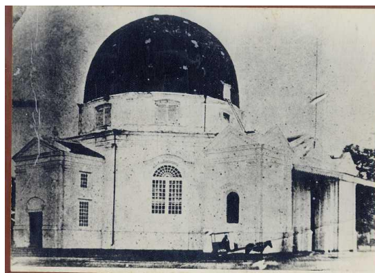
Figure 2. Blenduk Church Before the Conservation Source: Collection of Tropenmuseum, 1939
