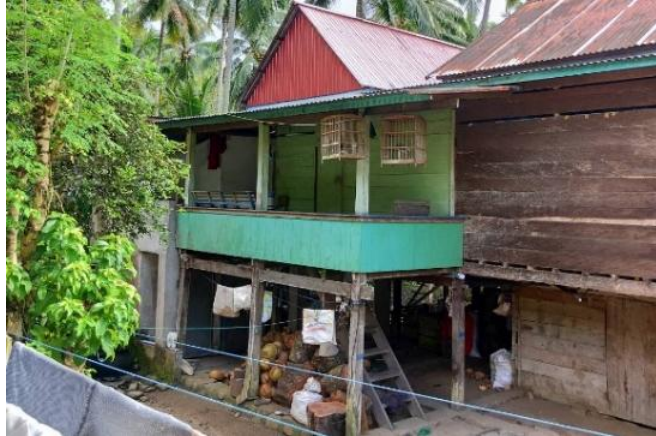
Figure 6. The Stairs and The Position of The Toilet (Outside the House) in Vernacular House
