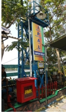
Figure 2. Waste Water Treatment in Kampung Sepoloh
