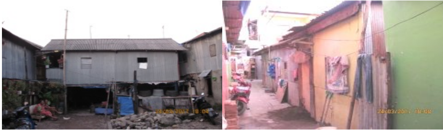
Figure 6. Physical Condition of Housing
