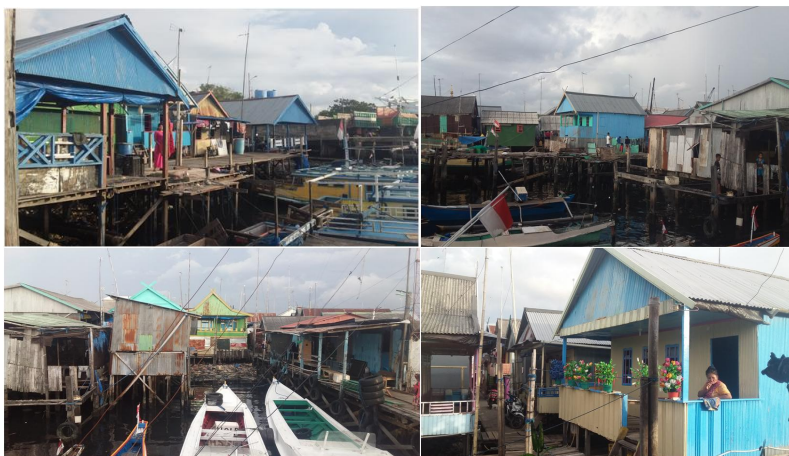
Figure 3. (Continuance) Physical Building Condition in Zone 1
