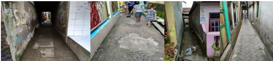
Figure 10. Physical Condition of Street
