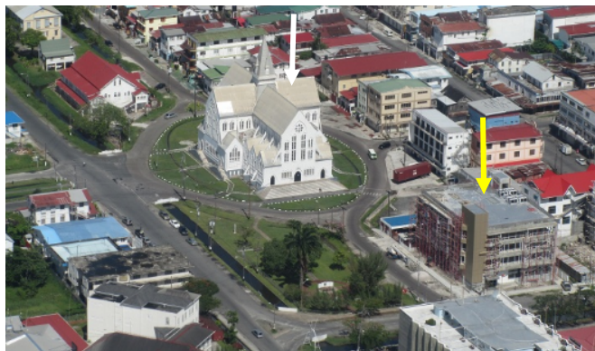
Figure 4. The New Building Society in Juxtaposition with St. George’s Cathedral and the Bank of Guyana
