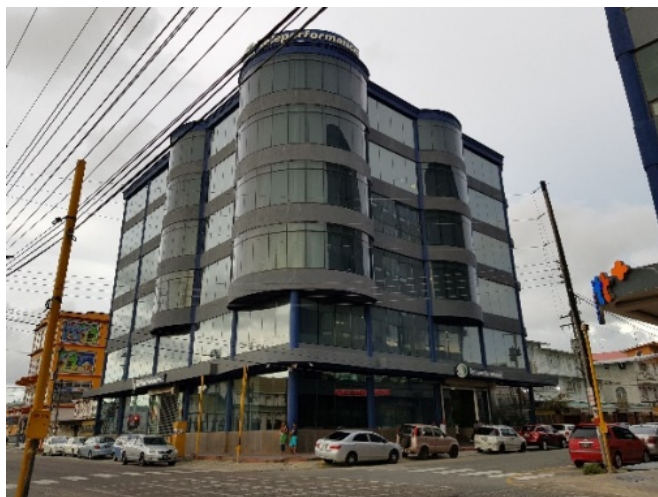
Figure 6. Telecommunications Office Source: Image Courtesy Yancey Haywood
