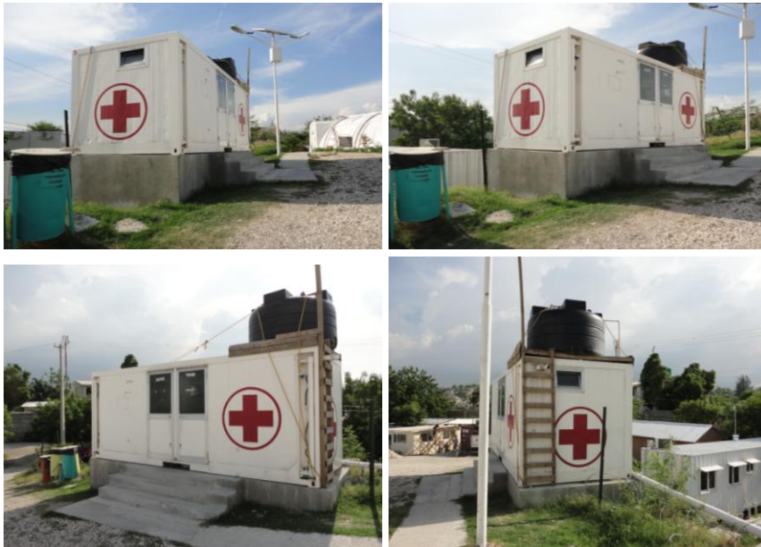
Figure 1. Input Photographs for Container Source: author's documentation
