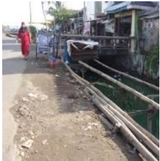
Figure 15. Raised Rack Frame Above the River Banks
