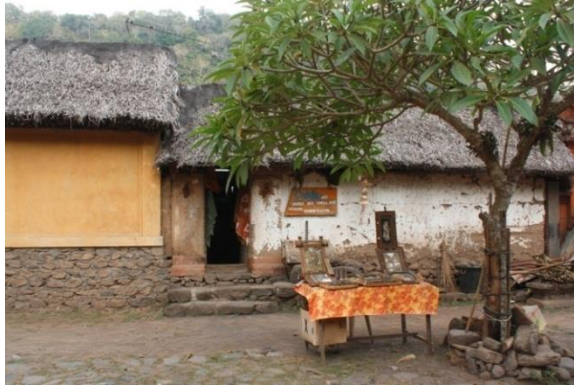
Figure 7. The Impact of Staggering Roof Form Source: field survey, 2013
