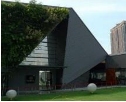
Figure 4. Lot 10 Roof Top, Bukit Bintang Source: field survey (2013)
