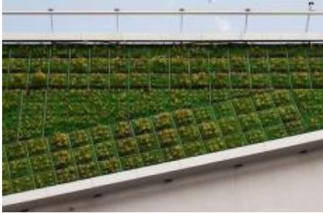
Figure 10. Digi Technology Operation Centre Apply Carrier System Source: field survey (2013)
