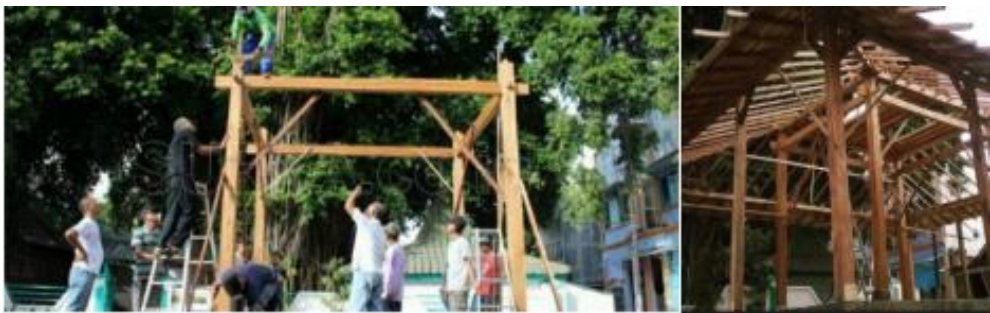
Figure 6. The Joglo Assembling Process (renovations, wood materials)
