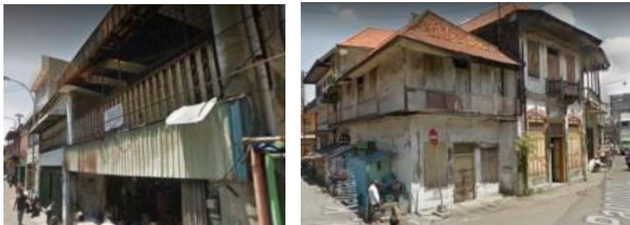
Figure 25 . Balustrade installed on the balcony terrace Source: google map
