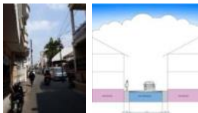
Figure 5 Large chunks of Road Ketapang Source: Personal Documentation
