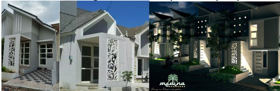
Figure 8 Secondary skin and shading device on the front of the building unit Medina Residence 1 (left), 2 (middle), and 3 (right) Source: Field Survey 2020
