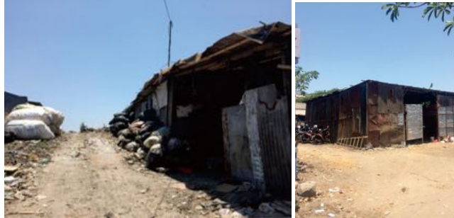
Figure 5. The Current Condition of Kampung Keputih Tegal Timur Source: Field survey (2018)
