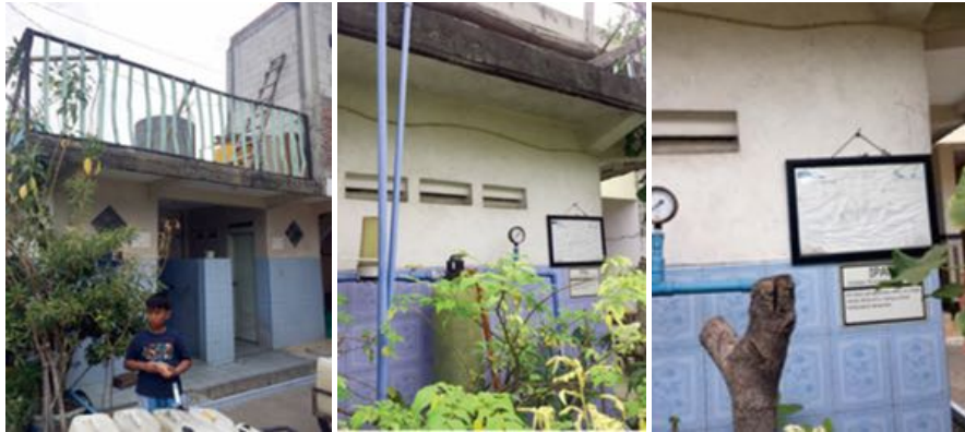
Figure 9. Public Facilities Centre for Water Distribution
