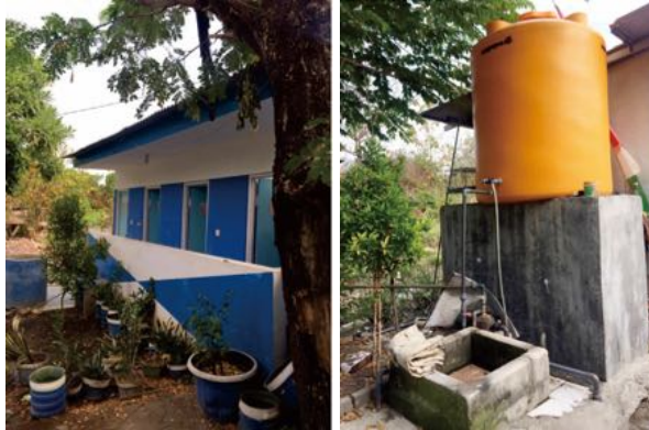
Figure 11. Public Toilet in Kampung Hijau Keputih Tegal Timur Source: Field survey (2018)
