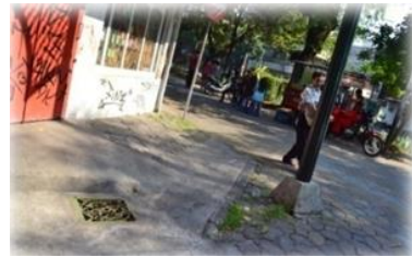
b. On type of drainage that flank the road, mounted control boxes to check and periodic maintenance of drainage channels.
