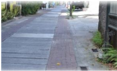
a. Circulation pathways in the Tourism Village Kauman using cast concrete with installation of porous so that water can get into the drainage channel in the middle, while the edge of the road there is infiltration area for environmental sustainability.
