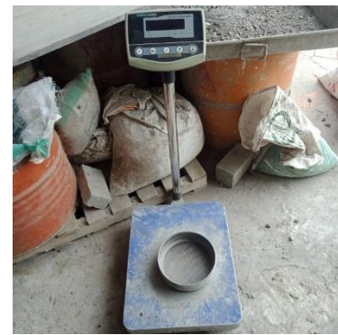
Figure 5. Concrete mix scale
