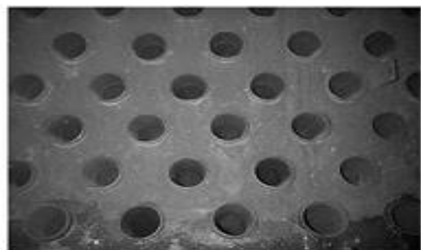
Figure 6. Visual inspection of boiler
