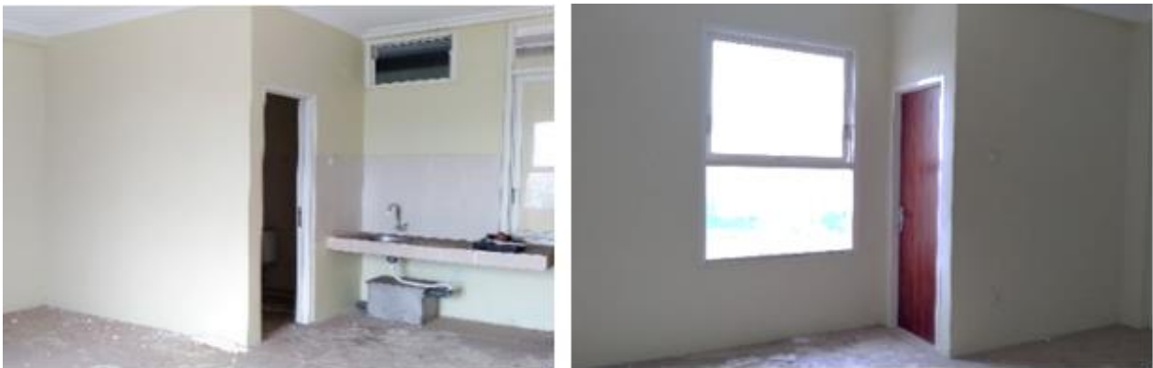
Figure 2. The interior of Rusunawa Siwalankerto 2.
