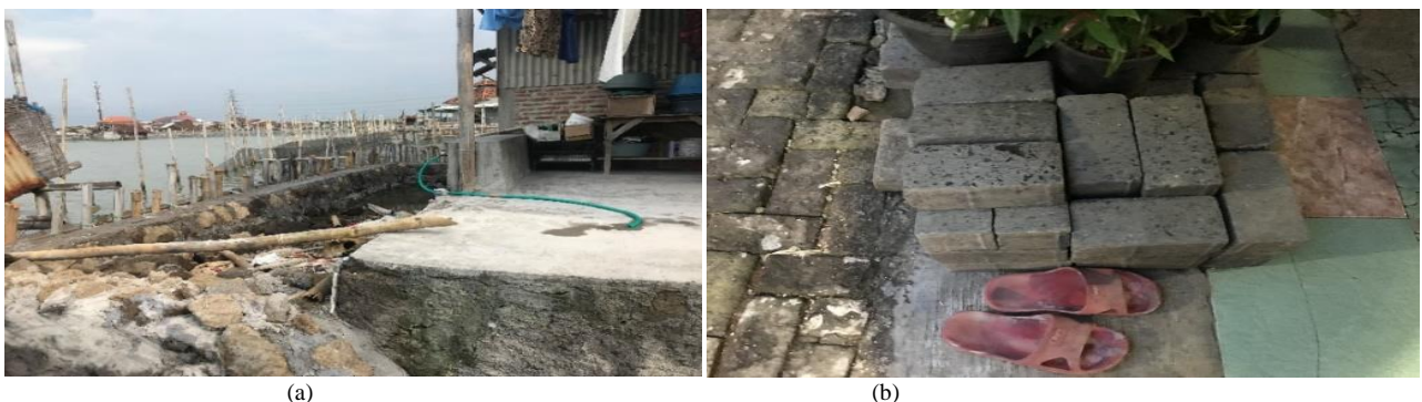
Figure 10. Condition of the house with adaptation (a) making embankment; (b) make a tidal flood barrier
