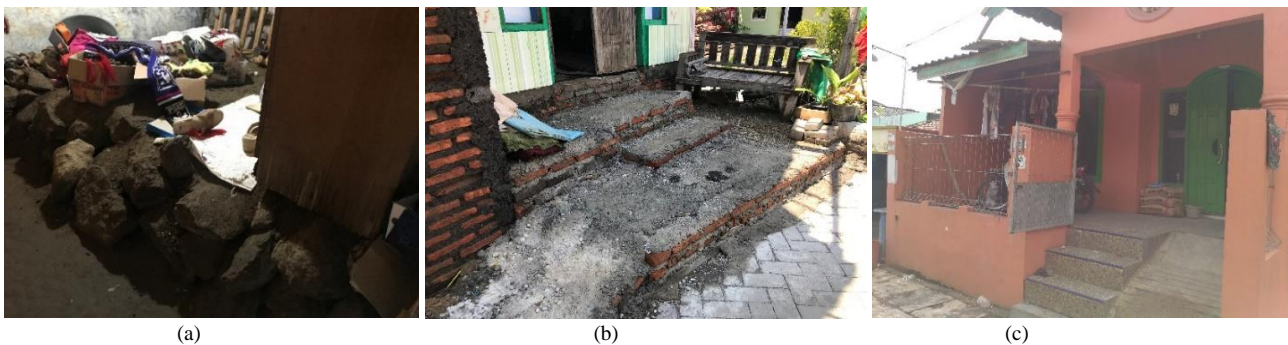
Figure 7. Condition of the house with adaptation (a) with landfill; (b) with plaster / cement / paving; and (c) with ceramic.
