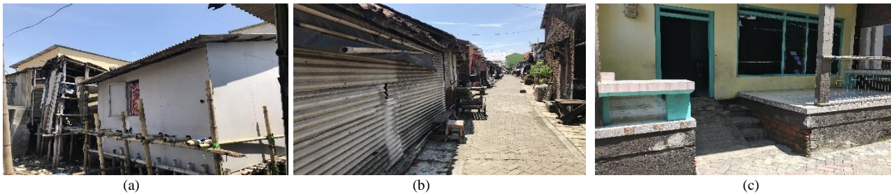
Figure 1. Housing conditions (a) non-permanent; (b) semi-permanent; and (c) permanent.
