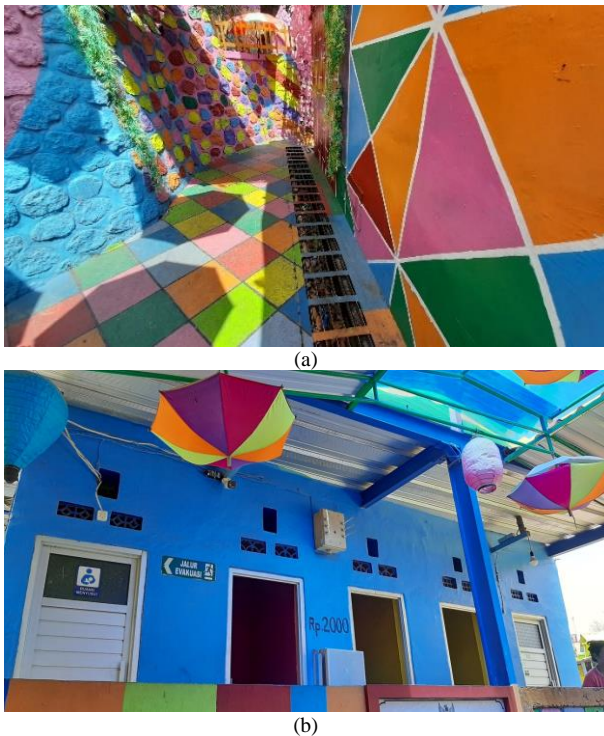
Figure 3. (a) Physical Condition of Drainage Channels; (b) Shared Bathroom in Kampung Jodipan.
