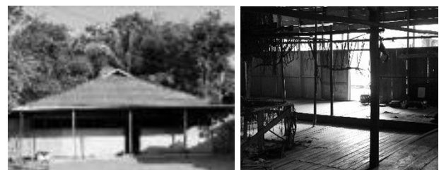
Figure 3. Daylighting Condition in Balalai Padang Adat House
