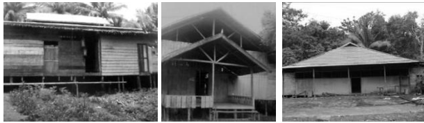
Figure 4. Balai Adat House. Bidukun Type (Left), Jalai Type (Centre) and Padang Type (Right)
