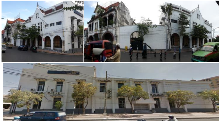
Fig. 11. Mandiri Building. (Researcher, 2016 and Google Earth )
