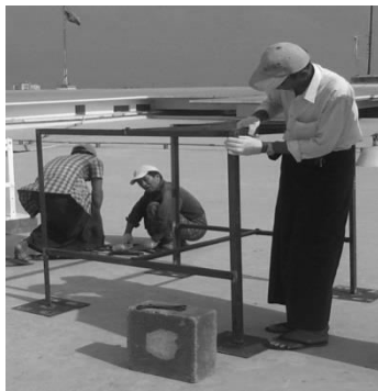
Figure 6. Construction of exposure rack
