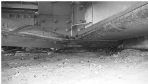
Figure 1. Moving Shoe of Bayinaung Bridge
