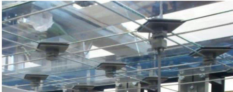
Figure 4. A pair of 75mm by 75mm of square plates used to clamp the glass to the cable network which fitted on top of the cable to cable clamp block.
