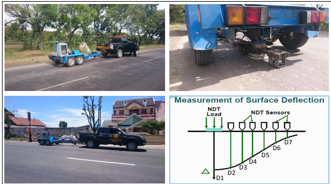
Figure 2. Testing activities during the pavement deflection measurement using the FWD apparatus.
