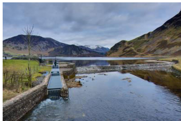
Figure 8 Ennerdale lake fish pass ( http://cumbria.unitedutilities.com )
