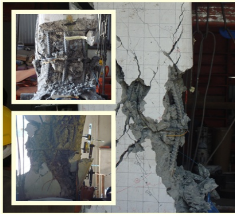
Figure 2. Failure of column specimen C-1
