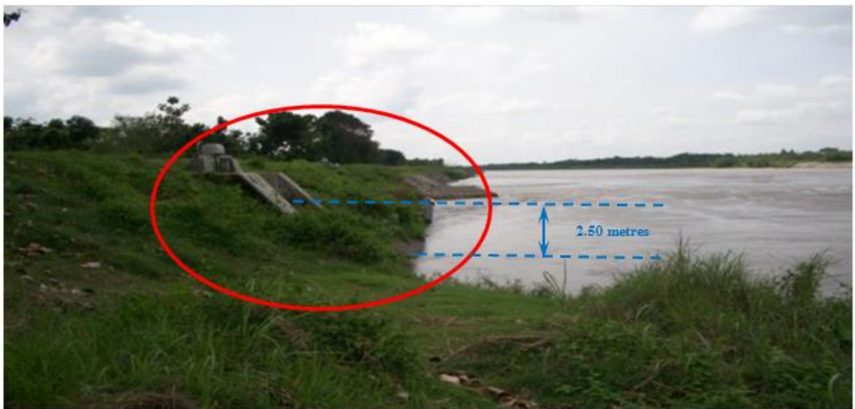
Figure 8. Water level below irrigation intake at downstream of Menturus rubber dam in June 2011
