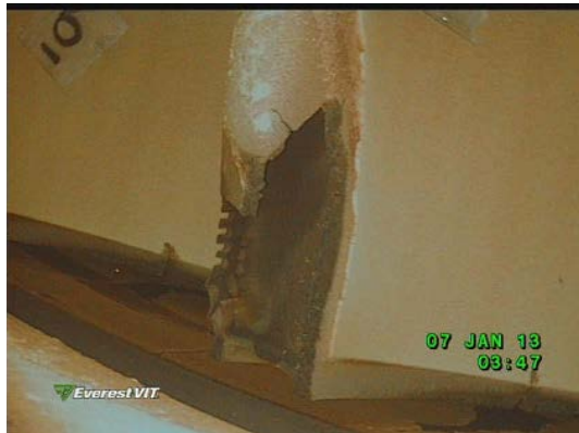
Figure 3. Missing Leading Edge.
