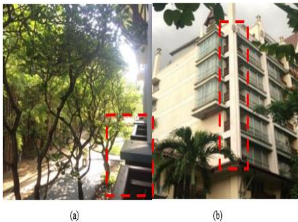
Figure 13. (a) The use of a Balcony at 3 floor building; (b) The use of a Balcony at 10 floor building.
