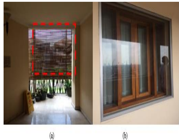
Figure 15. (a) Design of sun visor in Buildings; (b) Use two layers of glass.
