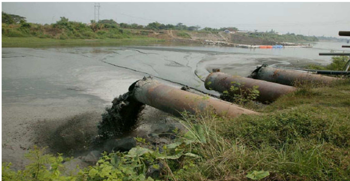
Fig. 6. The mud discharge channels to the Porong River (Kali Porong)
