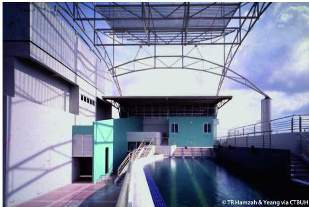
FIGURE 19 Evaporative cooling pool at Mesiniaga Tower.
