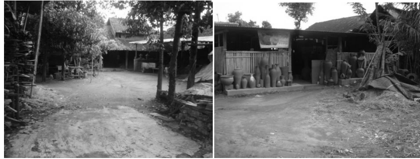
Figure 9. Latar is available even though the expansion tendency of showrooms and workshop area toward front yard become a common phenomena in Kasongan in 2012
